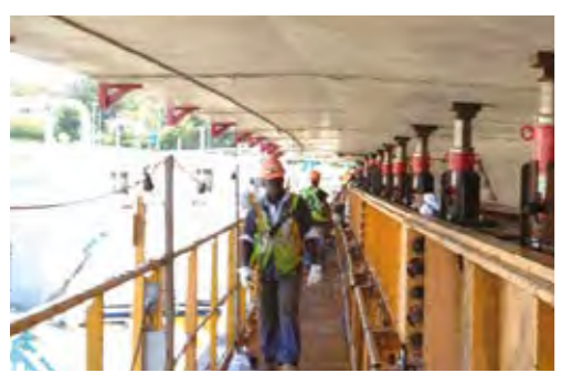
(42) HLN5508 lock nut cylinders lifting the Jordan Bridge in Chesapeake, VA.
